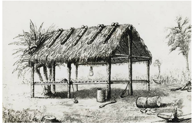
Figure 1. Minimally processed Cypress timbers and Palmetto thatch roofs used in the Seminole chickee huts. Image from MacCauley's report (MacCauley 1887) National Anthropological Archives, Smithsonian Institution, Neg. No. 1178-N-8-1.
